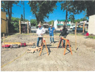
Ceremonial Garden Construction
